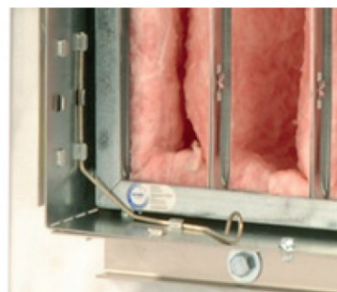
Universal Filter Holding Frame installation
